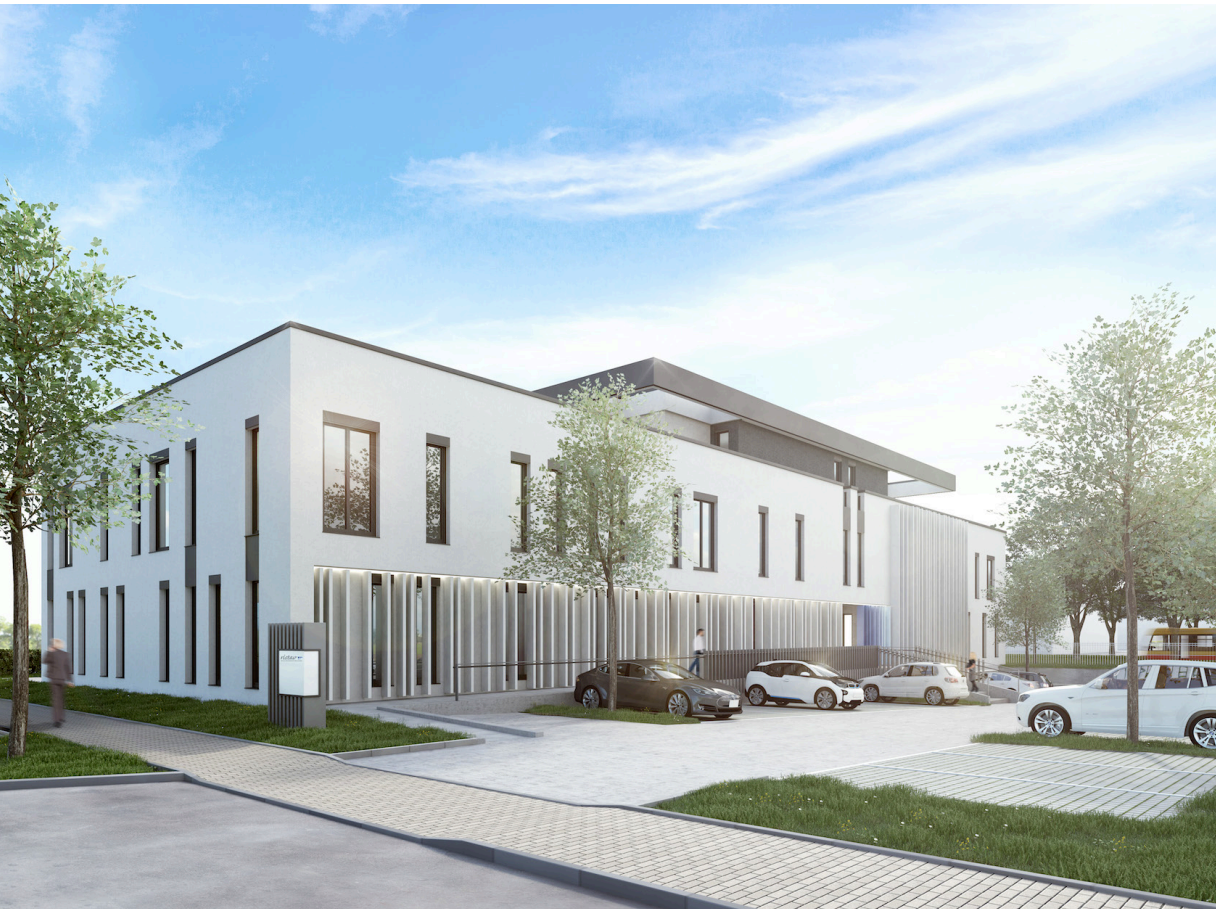
Project: ristav CUBE, Karlsruhe area, Germany
