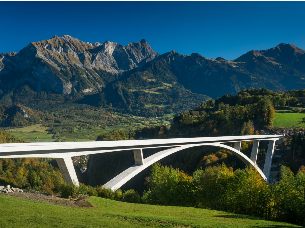
Tamina Bridge, Pfäfers Engineering office Leonhardt, Andrä und Partner, © Photo: Bastian Kratzke
